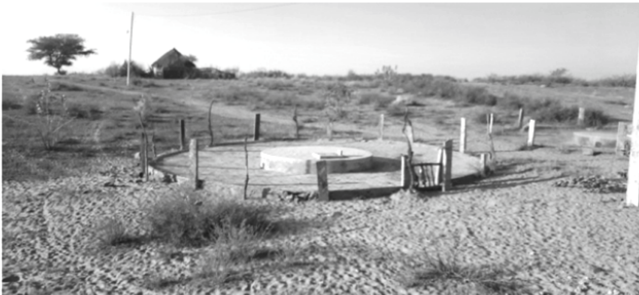
A taanka constructed in one of the project villages
